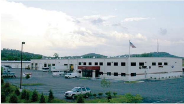
Modern Service Facilities...
